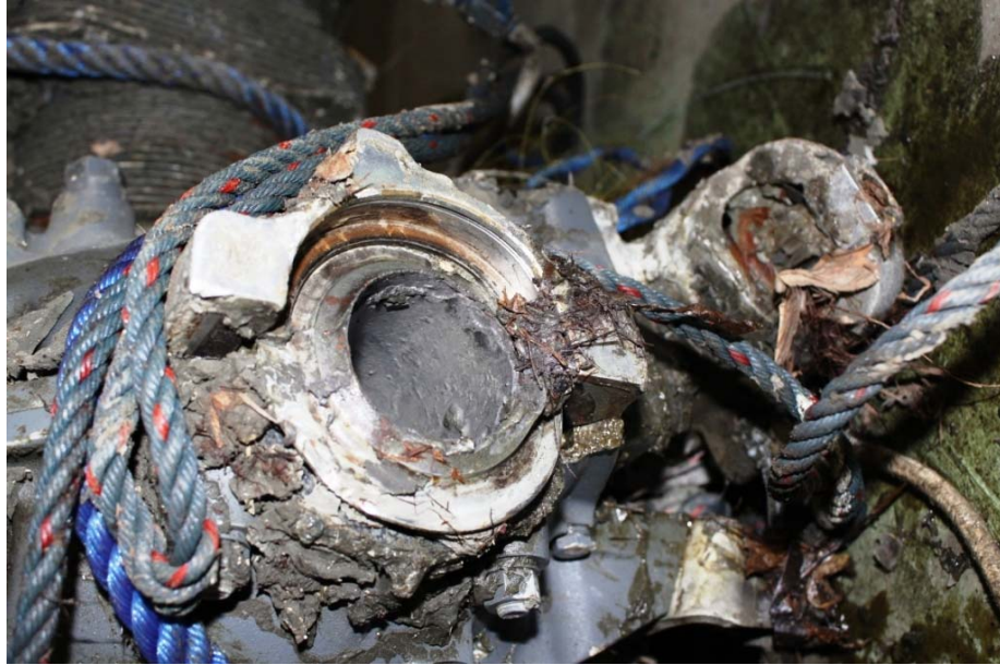
Figure 5: Broken propeller shaft
